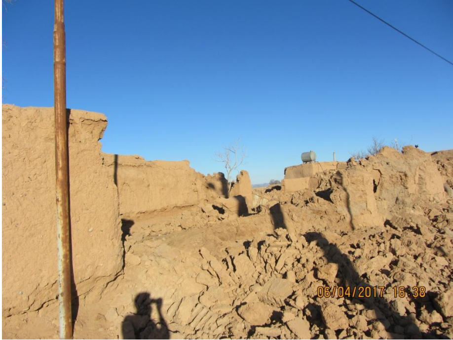
Figure 9. Demolition of farmhouse in the Doghalee village.
