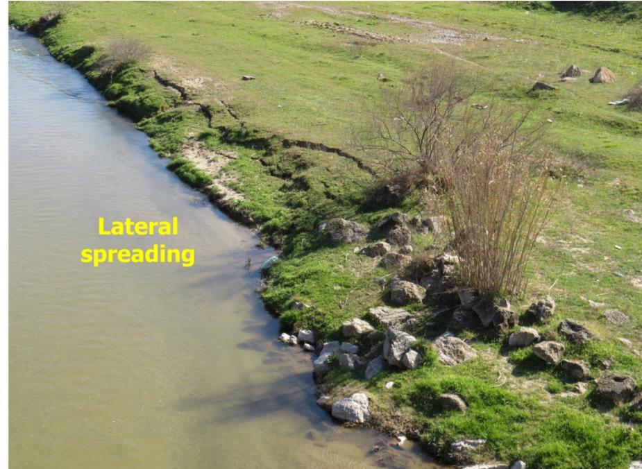
Lateral spreading along the banks of Titarissios River. The site is located downstream of the Damasi Bridge. It is significant to note that the Damasi bridge suffered heavy damage by the first earthquake. Thus, the authorities decided to temporarily close it for vehicles.
