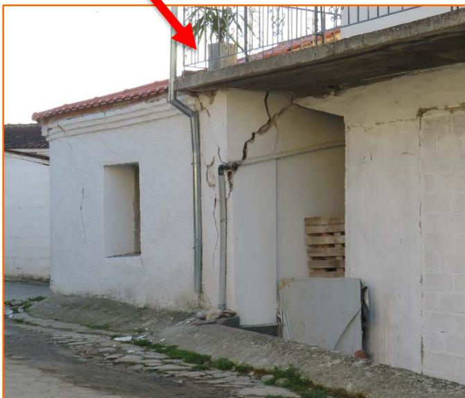
▲ Non-structural damage to building with RC frame and infill walls. It comprised detachment of plaster from the infill walls and extensive cracking of brick walls. The upper floor remained intact by the earthquake. The much softer ground floor is functioning as a kind of base isolator, absorbing thus, in its body, the seismic motion. The observed damage of the few partition brick walls is a physical consequence.
