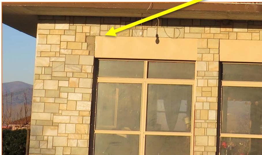
The majority of the reinforced concrete (RC) buildings of the earthquake affected area remained intact by the earthquake. Slight damage was observed to non-structural elements of the buildings. Typical example of slight damage are the detachment and fall of cornices, roof tiles and exterior wall cladding composed of different materials. We observed that the free standing or lightly anchored objects in stiffer structures suffered more damage compared to those standing in more flexible ones.
