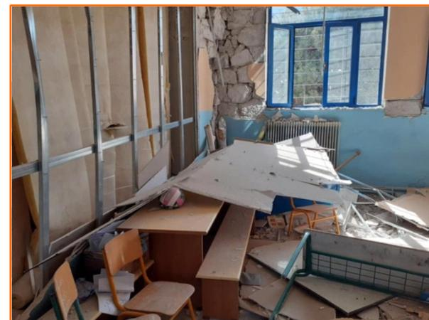
Views of the earthquake-generated building damage from the interior of the elementary school in Damasi village presented in the previous page. The masonry walls partially collapsed affecting only the school equipment.
