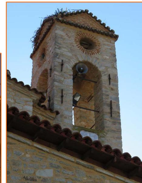
The seismic performance of churches depends on the geological formation of their foundation and on their strengthening. The church in Vlachogianni village remained untouched by the earthquakes. It is founded on alpine formations and moreover it has been reinforced with the installation of steel ties in the bell tower and in the other parts of the construction. The steel ties are placed in critical key points for the stability of the structure.
