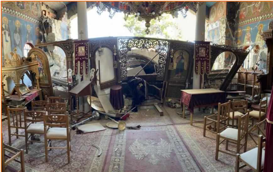
Partial and total collapse of the old and new masonry churches of Agios Nikolaos in Koutsochero village. The old structure completely collapsed, while the new one suffered collapse of its walls behind the altar.
