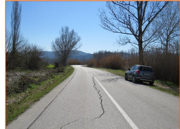
Damage to road leading from Mesochoiri to Vlachogianni was attributed to the earthquake ground motion and to the generated liquefaction phenomena affecting the area between the aforementioned villages.
