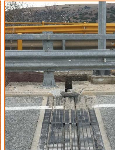
Pounding-induced damages attributed to the presence of these expansion joints were observed in several bridges in the earthquake-affected area. Pineios bridge close to Koutsochero Village is one of these examples.
