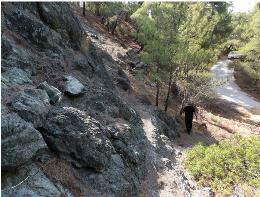
Figure 11: Partial views of the NW-SE striking and SW-dipping Polichnitos fault. It juxtaposes ophiolites in its footwall (left side) against Quaternary deposits (right side) in both figures.
